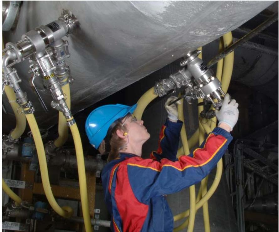
Wetend has developed a new concept where opposite charge chemicals or pairs of chemicals can be mixed in a single reactor zone with good results. The technology provides an opportunity to i.e. maintain generated filler-fiber composite and flock structures intact before forming and dewatering. It also enables the use of aggressive additives as well as develop composite structures for the web. This is
