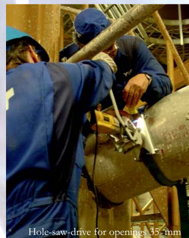
Hole-saw-drive for openings 35 mm
